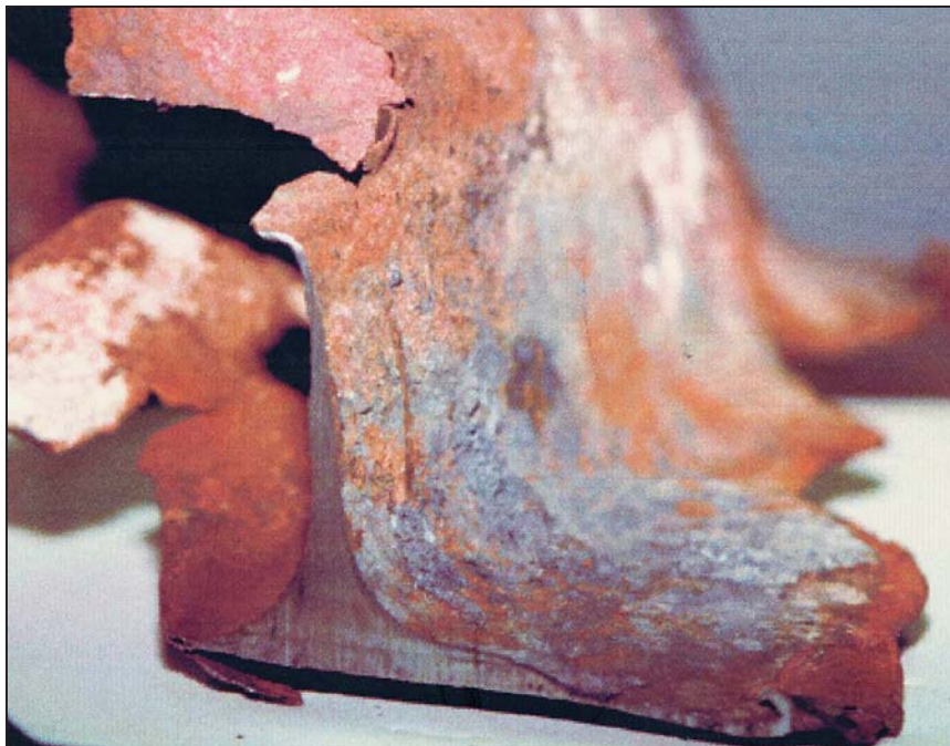
Figure C-2 Closeup view of eroded wide-flange beam section.
