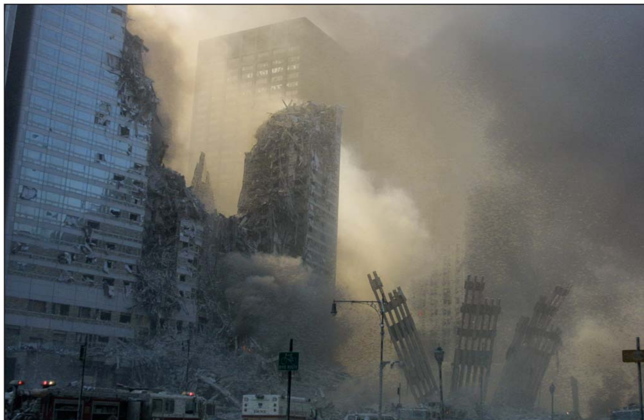
Figure 3-7 Partial collapse of WTC 3 after collapse of WTC 2.
