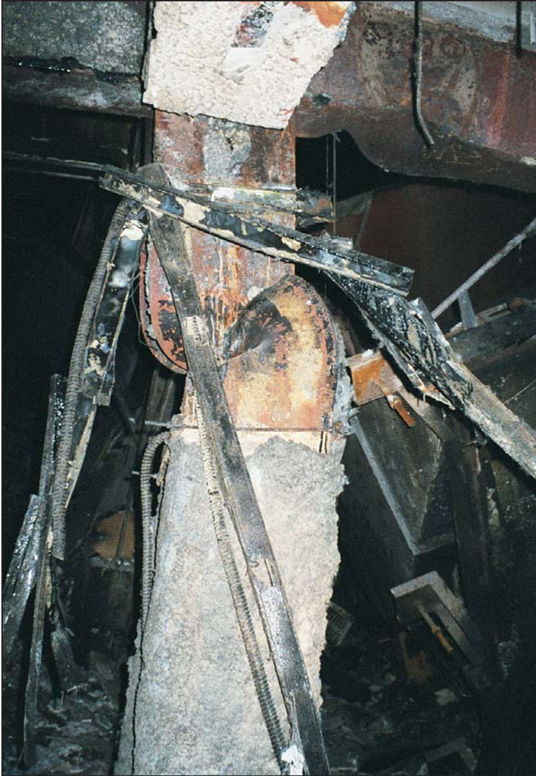
Figure 4-17 Buckled beam flange and column on the 8th floor of WTC 5 that was weakened by fire.
