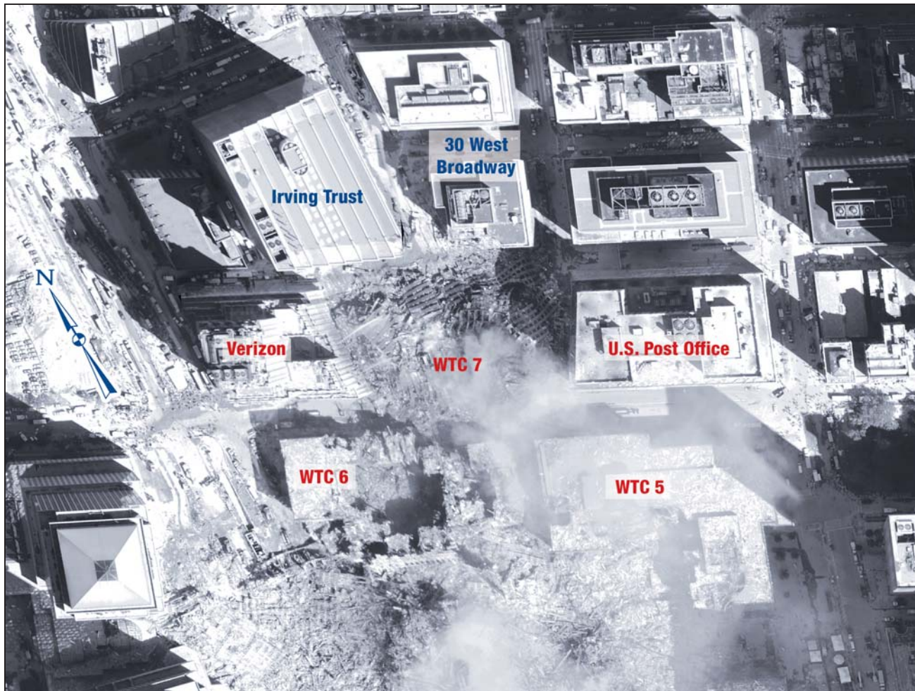
Figure 5-26 Debris generated after collapse of WTC 7.
