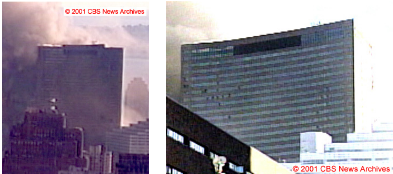
Figure 5–202. Cropped frames from the Camera 2 video clip in Figure 5–185 and the Camera 3 video clip in Figure 5–186, showing the north face of WTC 7 8.1 s \pm 0.1 s after the east penthouse began to move downward.
