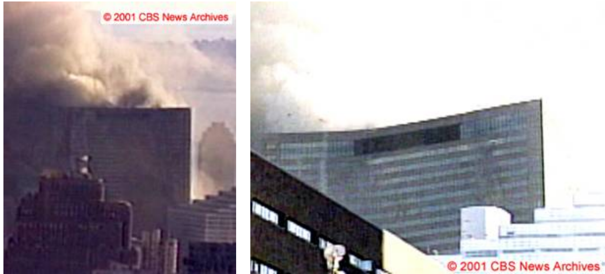
Figure 5–208. Cropped frames from the Camera 2 video clip in Figure 5–185 and the Camera 3 video clip in Figure 5–186, showing the north face of WTC 7 10.0 s \pm 0.1 s after the east penthouse began to move downward.
